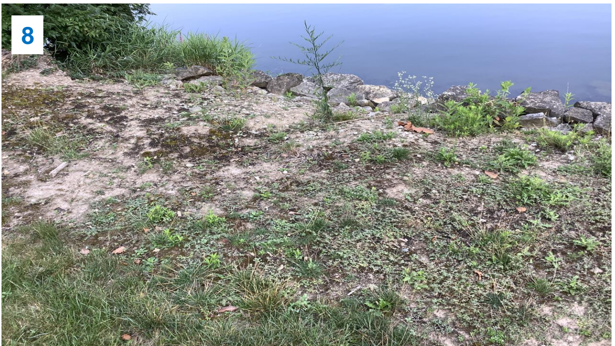
Top: Upstream slope on the left side, burrow holes by dock.
