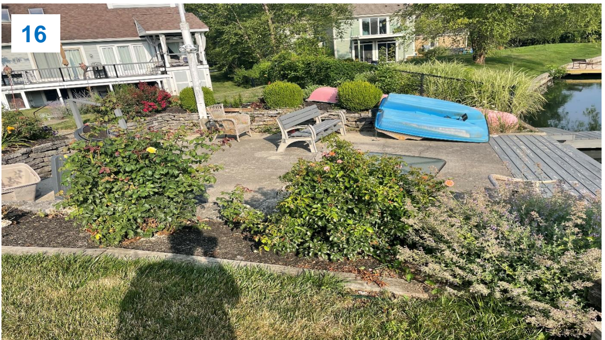
Top: Upstream slope right side, landscaping, fireplace, and garden on embankment.
