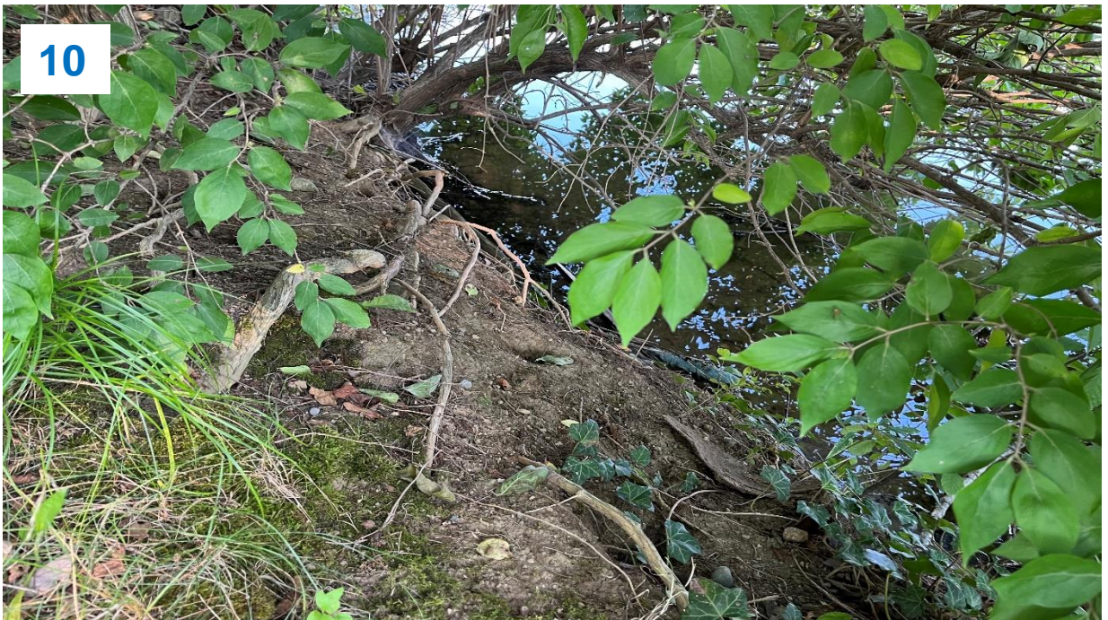
Top: Upstream slope on the left side, burrow holes near bush.
