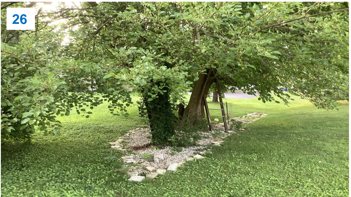
Top: Crest near right abutment, garden and vegetation with surrounding bare areas.
