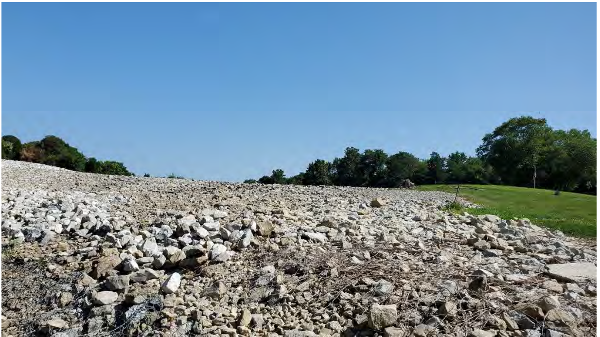
Top: Auxiliary spillway open channel. Note newly placed riprap.
